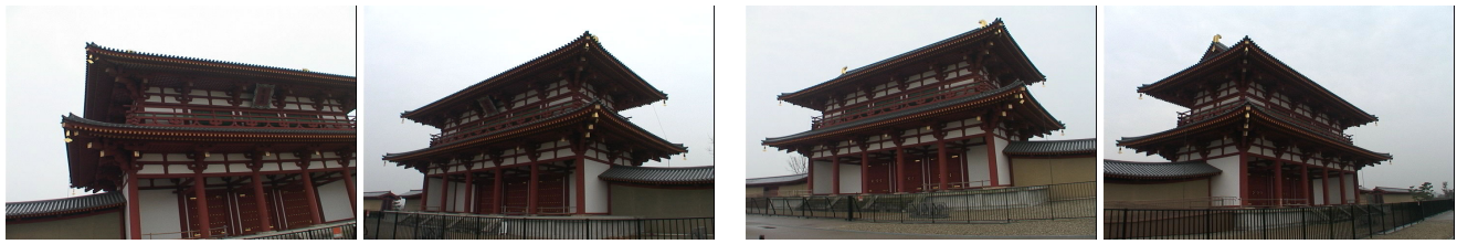
(a) front of building
