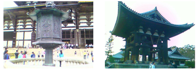
Figure 13: Photos whose shooting directions were similar to the directions of shooting positions to subject positions.
